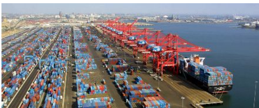
Figure-9: Container terminal, Long Beach, California, 2009
